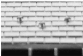
THESE ARE "SNOWBIRDS" THAT WERE USED ON ROOFS TO KEEP SNOW AND ICE FROM SLIDING OFF. MOLDED IN GRAY STYRENE.
