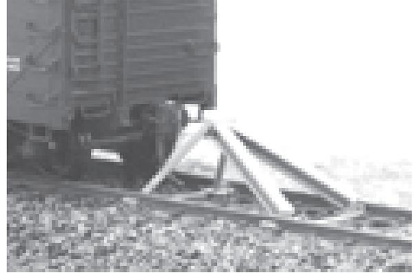
THIS IS A STANDARD HAYES MANUFACTURING CO. CAR BUMPING POST. IT WAS FIRST MADE IN 1926 AND CONTINUES IN USE TO THIS DAY. IT IS THE MOST COMMON TRACK STOP AND WAS USED ALMOST EVERYWHERE. THE KIT IS MOLDED IN GRAY STYRENE AND INCLUDES THE REINFORCING PLATES PLACED ON THE OUTSIDE OF THE RAILS.
